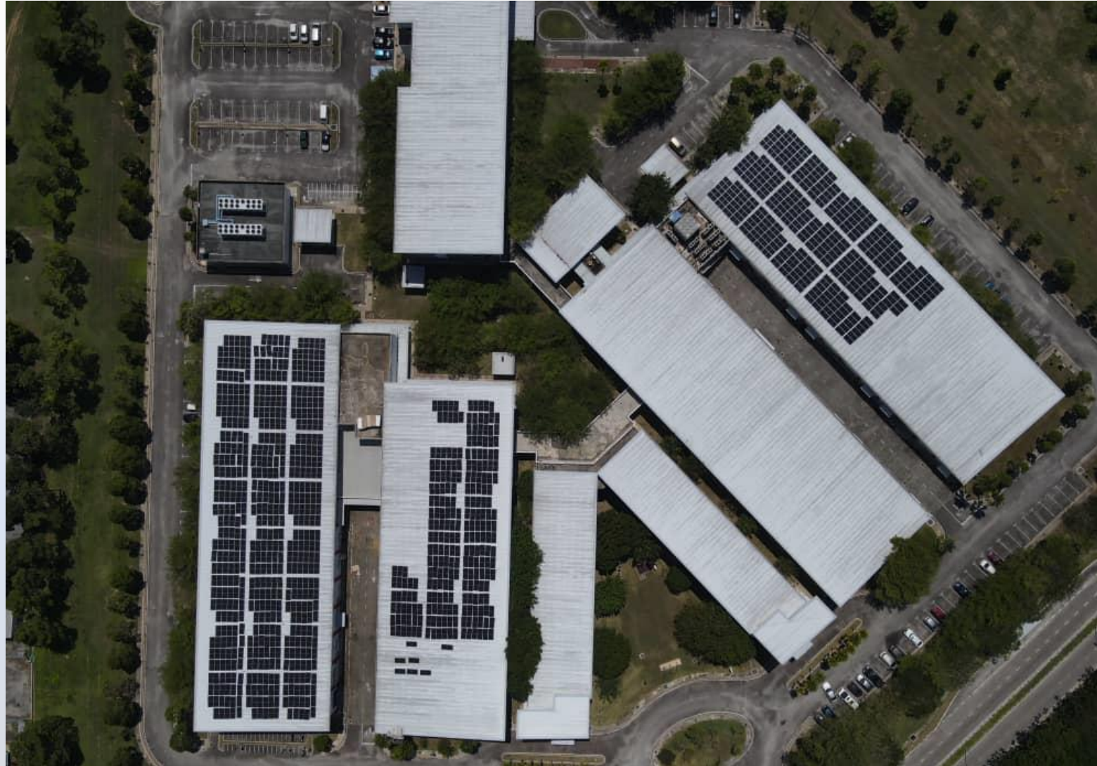
Picture of Roof and Solar Modules at FKP as of June 27, 2023
