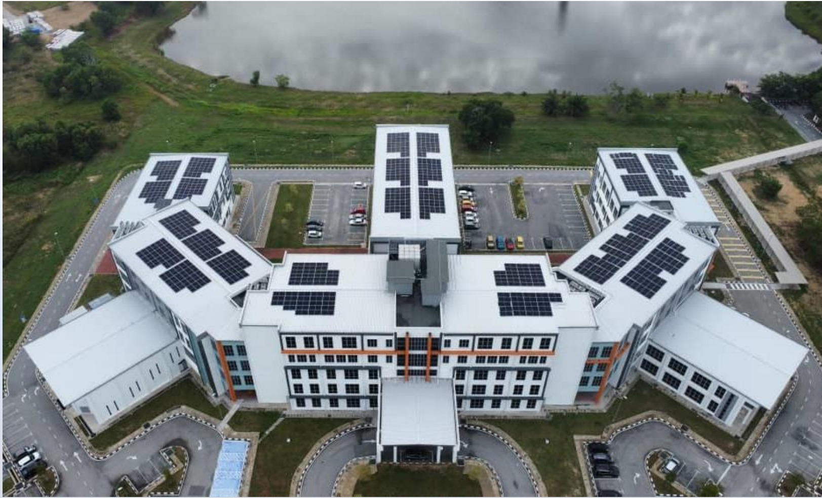
Picture of Roof and Solar Modules at FKOM as of June 27, 2023
