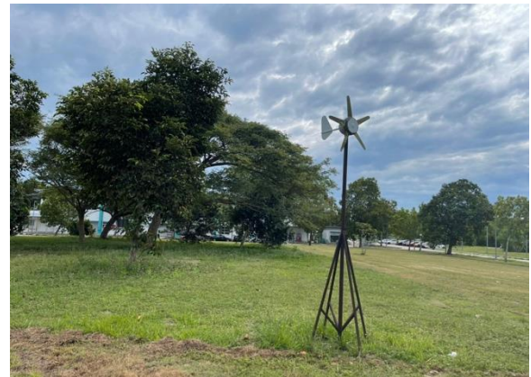
800W wind turbine at FTKMA
