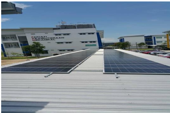
20kW Solar Panel installed on the walkaway roof at FTKMA
