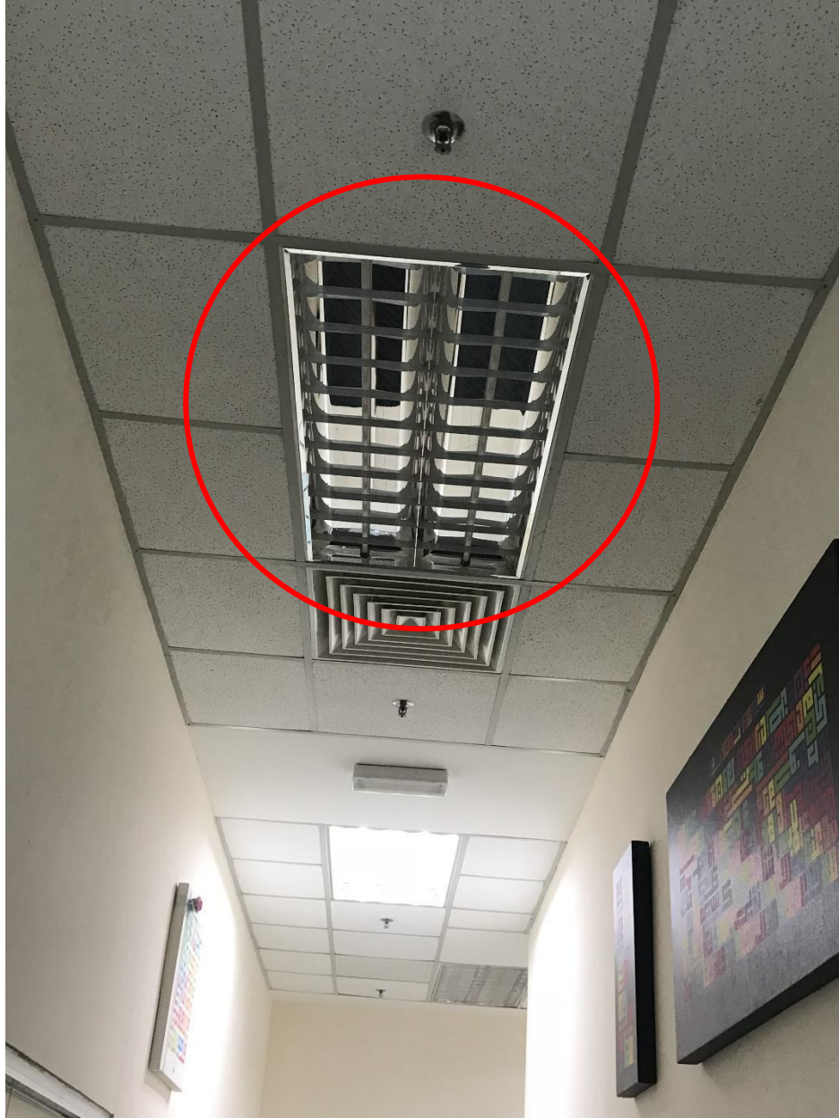
T8 florescent tube replace to T8 LED tube
